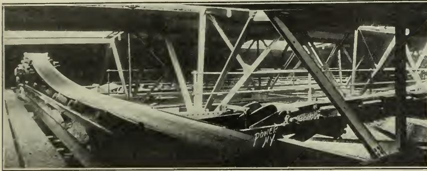
FIG. 10. COAL-CONVEYING SYSTEM ABOVE BUNKER
